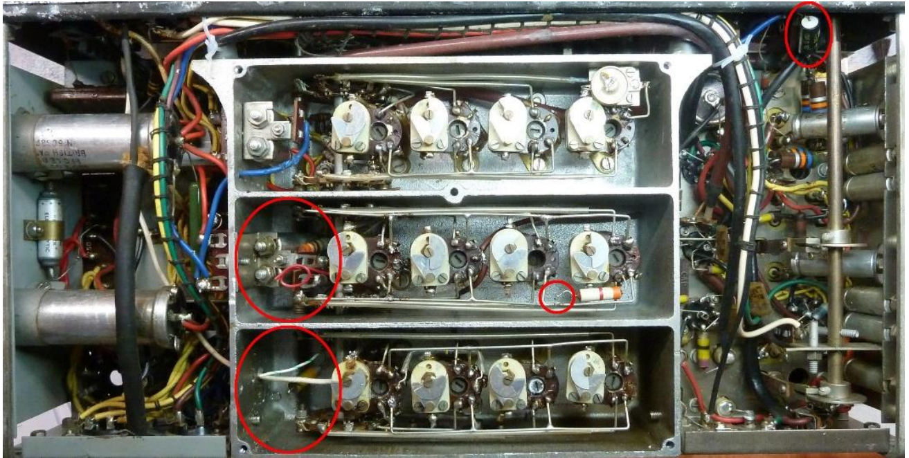
Figure 3: Chassis wiring of Eddystone S.750
