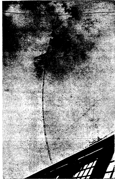
Fig. A. Showing Crossfeeder Aerial System in use at Eddystone Works.
