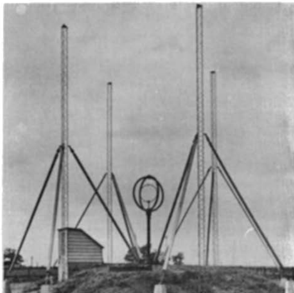
Cathode-ray direction-finding installation:
